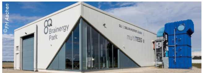
Heat storage device in front of the TESS 2.0 building in which the OTTOJUNKER Power-to-Heat system is integrated.
